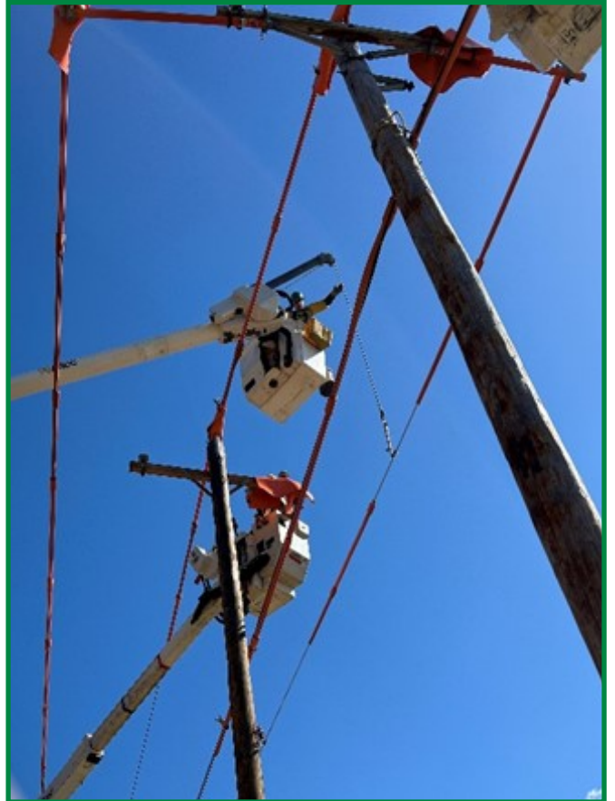
Pictured are employees of Delaware County Electric Cooperative and Steuben Electric Cooperative work together to safely move energized conductors to a newly set pole.
